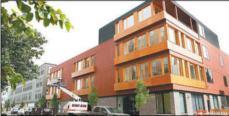
At 321-323 West Second St. in South Boston, Utile Inc. created a low, wide building inspired by nearby warehouses, the same concept used at the Trolley House next door (left). (Photos By Pat Greenhouse/Globe Staff)
